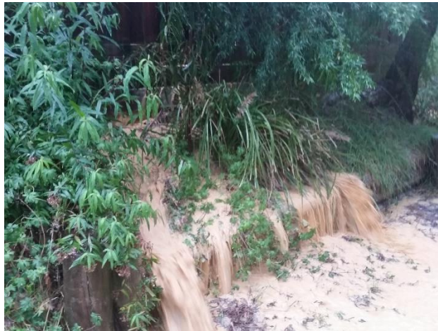
Figure 18 Run-off from a construction site adjacent to Valley Reserve which directly entered Valley Creek and the Regent St Wetlands.
